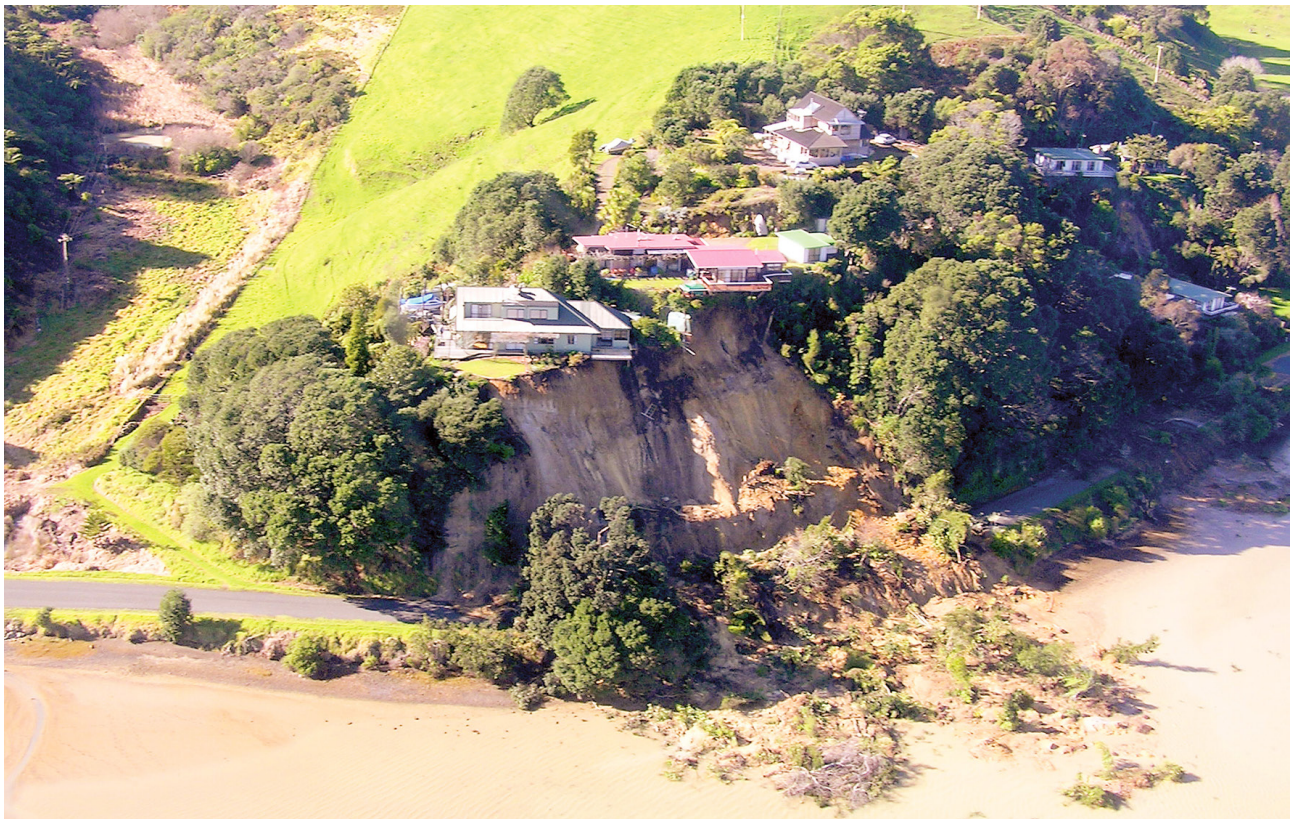
Eastern Bay of Plenty Landslip 2004
